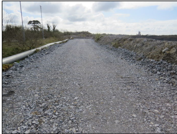
Plate 6.2: Spoil and bare ground habitat within the application site.
